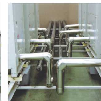
Existing piping reused from the base of the outdoor unit.
