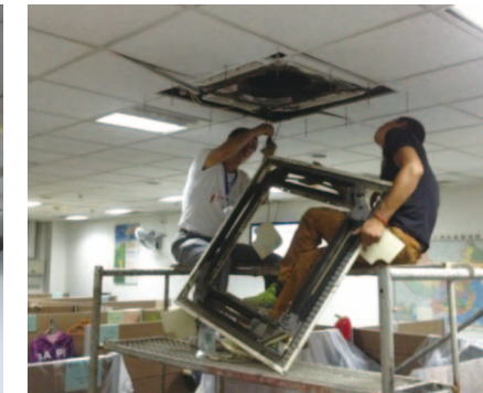
2 Removing indoor unit
