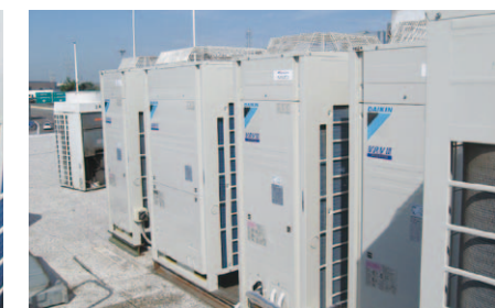
The VRV III-Q units run on R410A, ensuring compliance with the latest standards.
