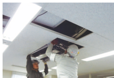
Removing old indoor unit
