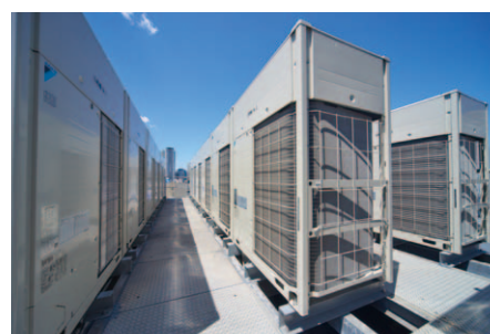
VRV Q installation
