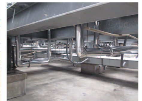
6 Refrigerant pipes under outdoor unit
