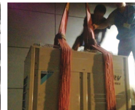
5 Installing outdoor unit
