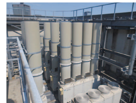
4 Existing outdoor unit. Based on airflow analysis, the discharge boot was decided to be removed. This realized a reduction of initial cost.
