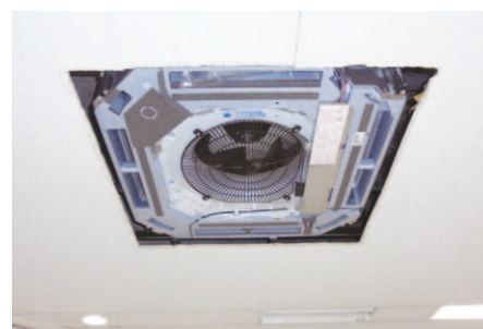
New indoor unit installed
