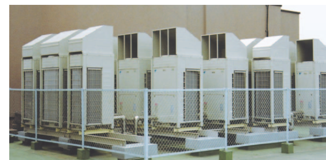
Reused existing foundation and replaced outdoor unit sequentially.
