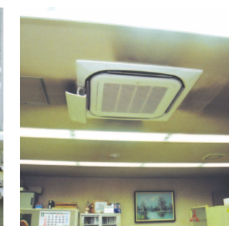
Installed round-flow type indoor units to every room without disturbing working hours.
