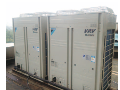
9 New VRV Q installation
