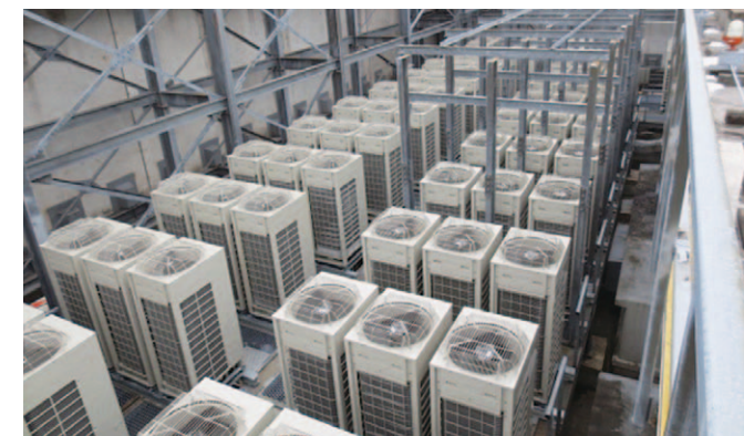
7 New outdoor unit installation
