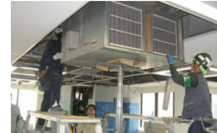
2 Removing existing indoor unit
